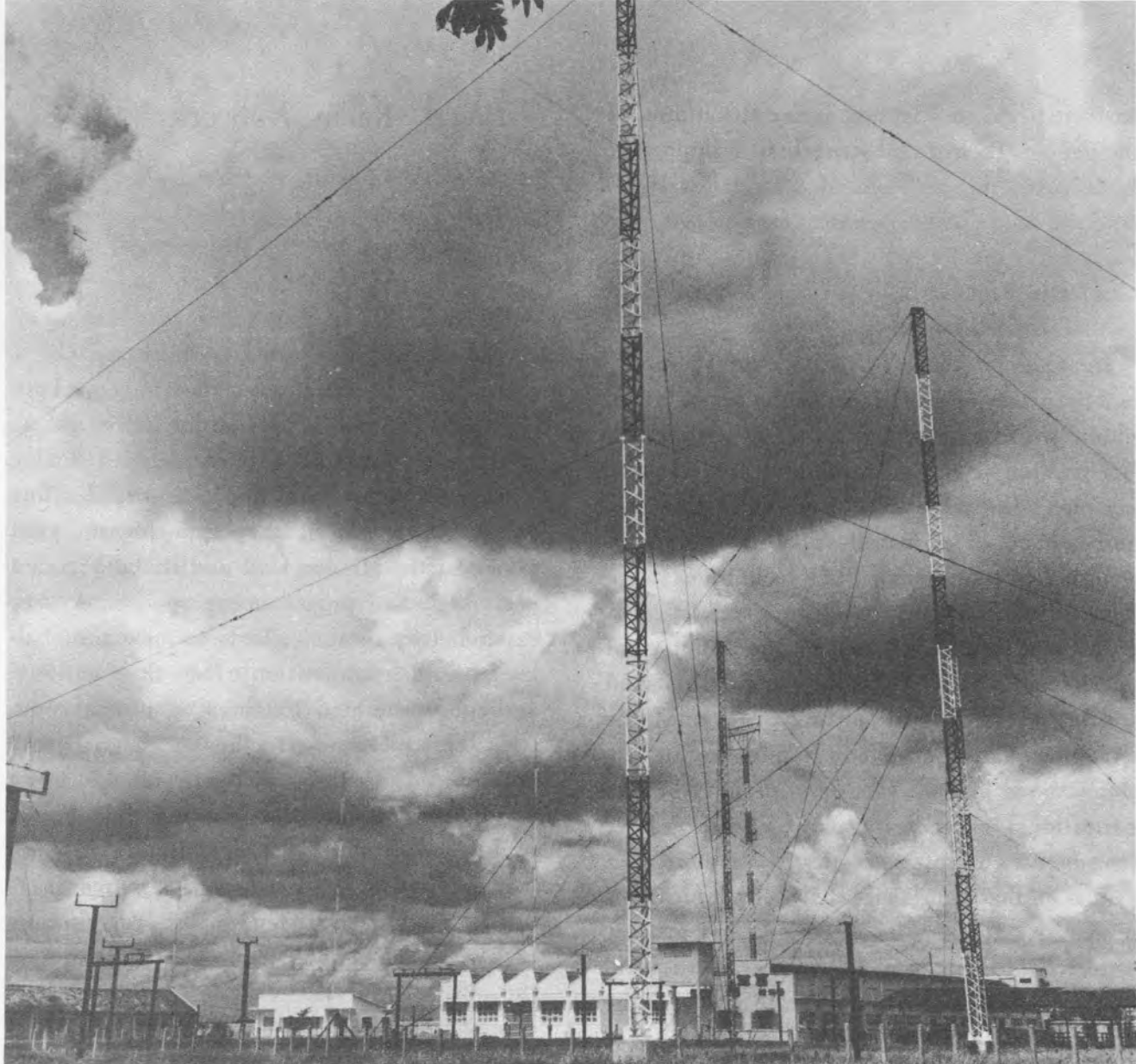
Quantre transmitting site at Saigon. Buildings house short and medium-wave transmitters – SW antennas in foreground and directional antenna in background.
