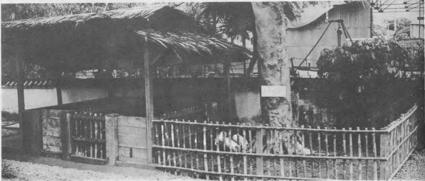
Cement has been provided by USOM to farmers for use in constructing pig-sties and compost shelters.
