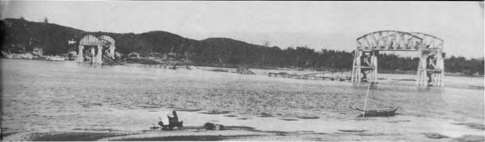
Route # 1, Km. 1055.5 - Quang Ngai. 640 meter, original structure completely destroyed, service provided by causeway and pontoon bridge; new bridge scheduled for completion July 1965.
