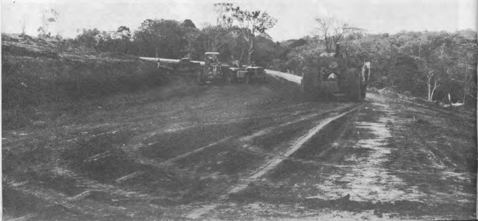
Equipment working on National Route No. 14.
